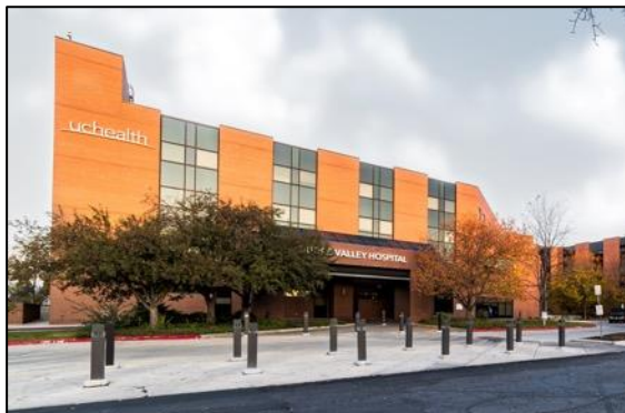
Poudre Valley Hospital
