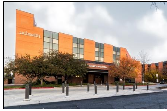
Poudre Valley Hospital
