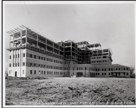
1938 Fitzsimons Building 500 Construction
